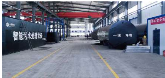
1. Integrated Sewage Treatment Equipment Production Workshop
