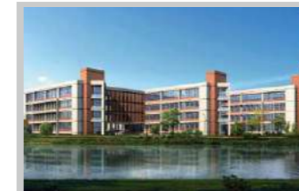
School domestic sewage treatment
