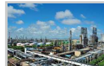
Domestic sewage from industrial enterprises
