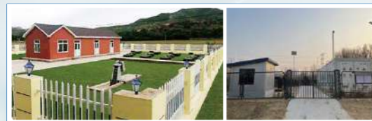
1. Third-Party Operation and Maintenance Services for Sewage Treatment Stations
